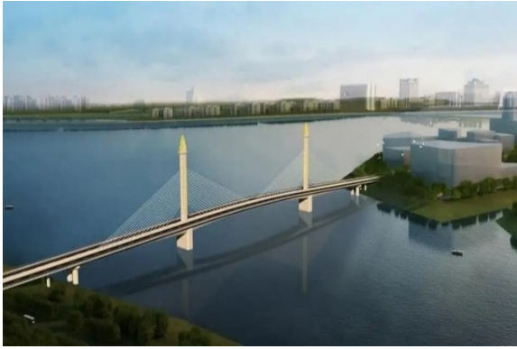
Phnom Penh's first cable-stayed bridge project
