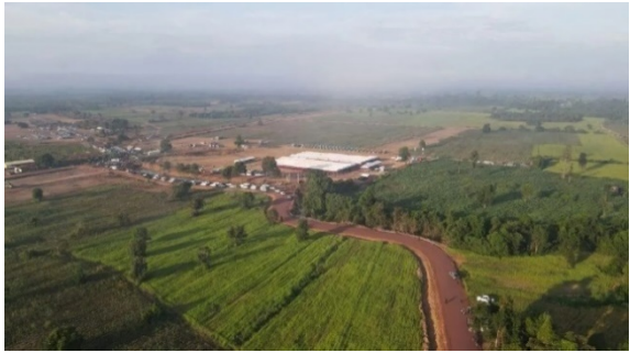
New Siem Reap's ring road projects worth $140 million
