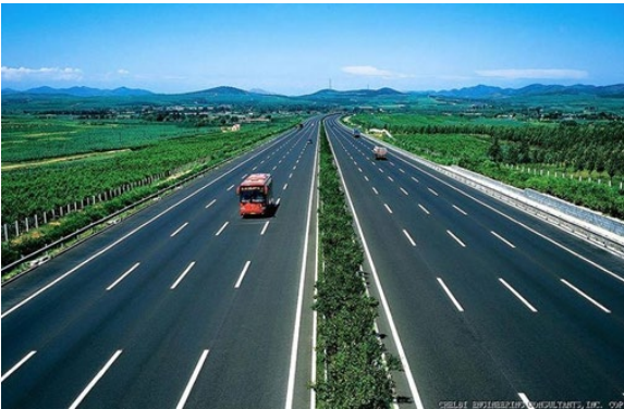
Construction of PP-Bavet expressway set to begin for June 2023
