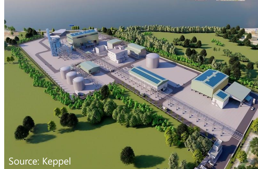
Keppel Sakra Cogeneration Plant (KSC Plant)
